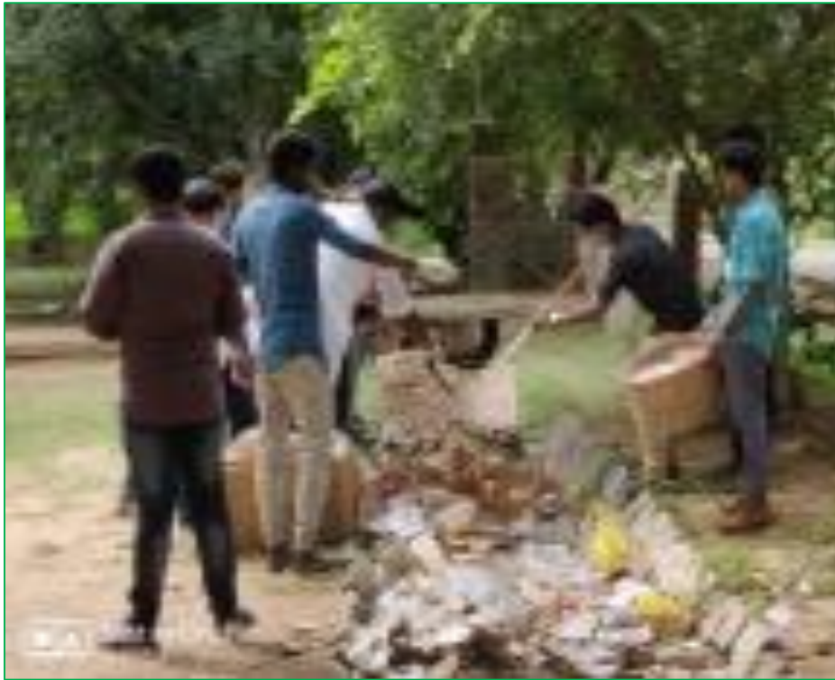
Cleaning work done at OFT Market on 21.09.2019.
