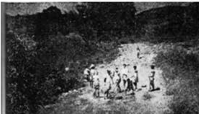
Laying a Road for progress at Pachaimalai
